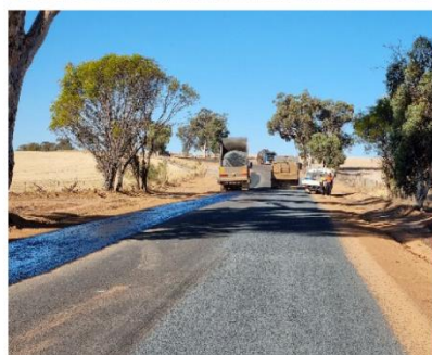
Shoulder widening Above: Bullock Hills Road Above Left: Beaufort Road Left: Beaufort Road
