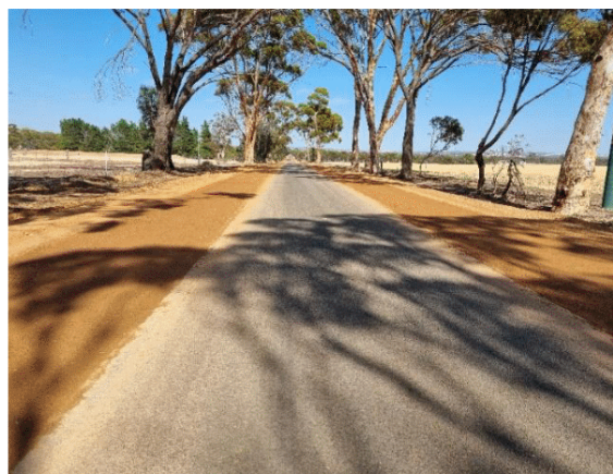
Shoulder stabilising in progress on Bullock Hills Road.
