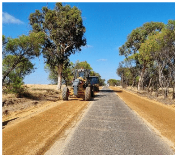
Shoulder stabilising in progress on Beaufort Road.
